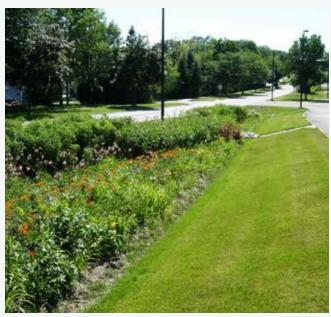
Bioswales are linear stormwater management systems that infiltrate, slow, and clean water when it rains
